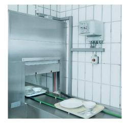
**Fire protection closure:** If the border of a fire compartment runs between the dishwashing area and the dining room then a fire protection closure must be provided.
