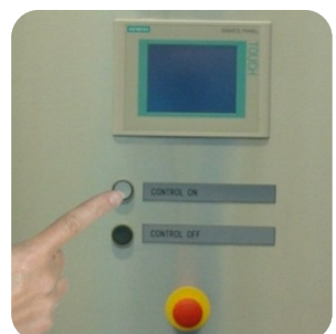
Press the "Control On" button on the switch cabinet. This automatically acknowledges emergency stop.
