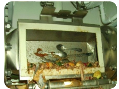
Open the pipe magnet and remove metal parts. Check the seal is clean and remove any dirt before you close the flap.
