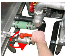
After you have installed the parts, close the open drain valves.
