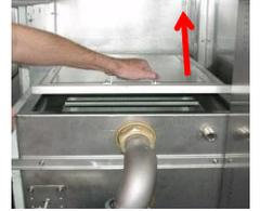
Remove the covering at the wash tank.
