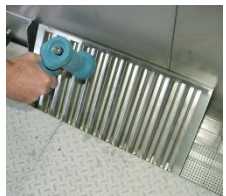
Clean the condensation separator.
