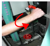
After you have installed the parts, close the open drain valves.
