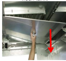
Remove the upper covering sheet.
