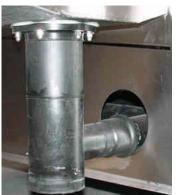
All discharge pipes for water from the machine must be connected to the kitchen waste water system via an adequately dimensioned odour trap.
