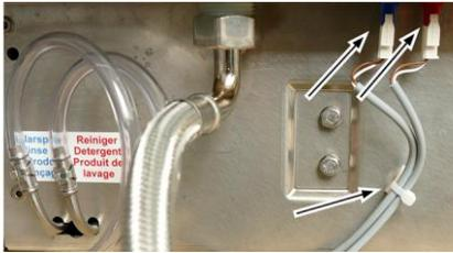
3. Insert the rinse aid and detergent suction lance plugs (blue or red label respectively) into the corresponding color-coded connection sockets.
