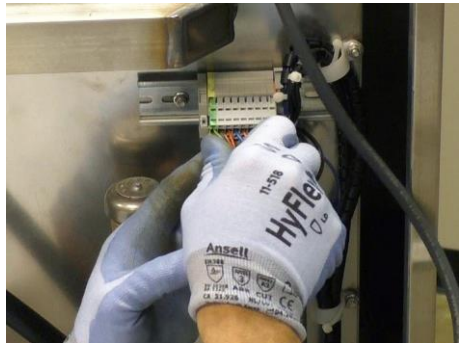
26. Press the plug into the top row of the connection block until it snaps into place.
